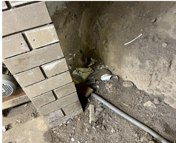
Line ID 84: Internal, Student Lodges, Blacksallees Lodge, Basement Plant Room, Adjacent Brick Pillar, Compressed Cement Sheetting Debris - Chrysotile Asbestos Detected
