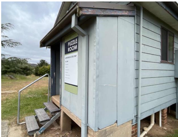
Line ID 46: External, TAFE, Classroom Building, Puzzle Room, Wall Panels, Fibre Cement Sheet - Chrysotile & Amosite Asbestos Detected
