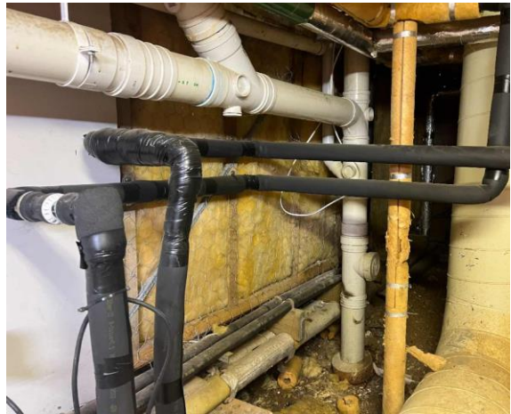
Line ID 199: Internal, Student Lodges, Snowgums Lodge, Basement Plant Room, Wall Lining, Insulation Batts - Suspected SMF
