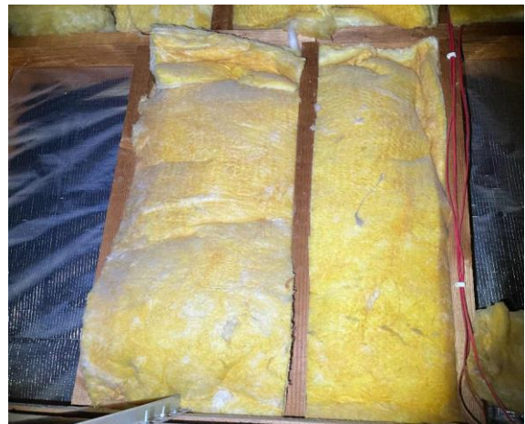
Line ID 166: Internal, Margin Lodge, Ceiling Void, Wall and Roof Lining, Insulation Batts - Suspected SMF
