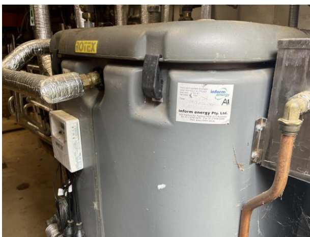
Line ID 184: Internal, Student Lodges, Kareela Lodge, Basement Plant Room, Hot Water Unit, Insulation Material - Suspected SMF
