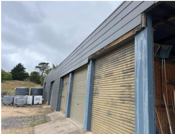
Line ID 52: External, Workshop, Roller Door Area, Wall Panels, Fibre Cement Sheet - Chrysotile Asbestos Detected
