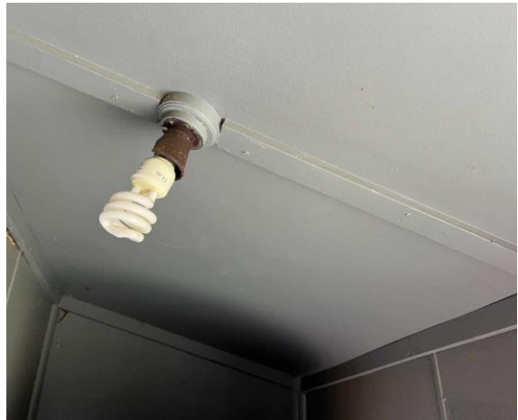
Line ID 45: External, TAFE, Classroom Building, Puzzle Room, Ceiling Lining, Fibre Cement Sheet - Chrysotile & Amosite Asbestos Detected
