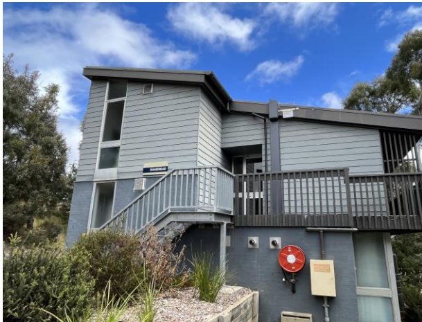
Line ID 36: External, Student Lodges, Ramshead Lodge, Outer Walls, Weatherboard, Fibre Cement Sheet - No Asbestos Detected
