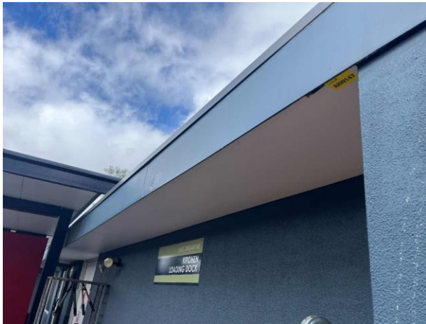
Line ID 4: External, Dining Hall, Loading Dock for Kitchen, Eaves and Fascia, Fibre Cement Sheet - No Asbestos Detected
