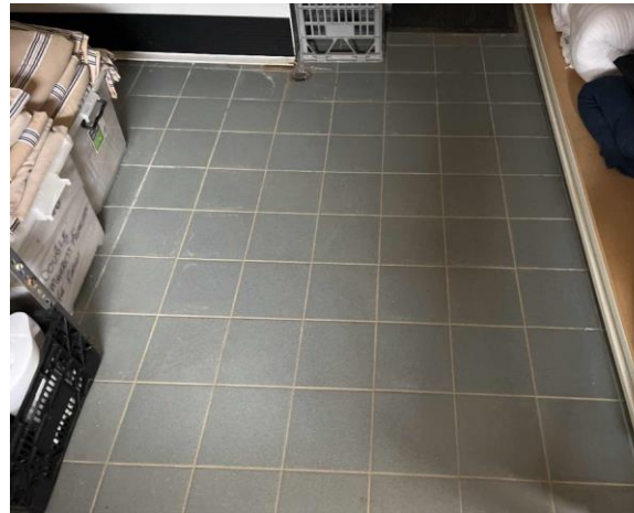
Line ID 64: Internal, Maintenance, Laundry, Below Ceramic Tiles to Floor, Compressed Cement Sheeting - Suspected Asbestos
