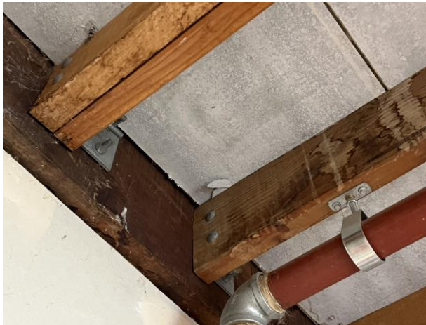
Line ID 86: Internal, Student Lodges, Blacksallees Lodge, Basement Plant Room, High Ceiling Lining, Compressed Cement Sheetting - Chrysotile Asbestos Detected
