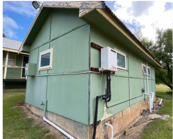
Line ID 17: External, Lodge 5, Toilet Block, Wall and Eave Linings, Fibre Cement Sheet - No Asbestos Detected
