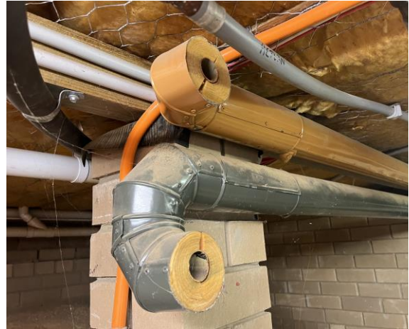
Line ID 189: Internal, Student Lodges, Merritts Lodge, Basement Plant Room, Pipes, Insulation Material - Suspected SMF
