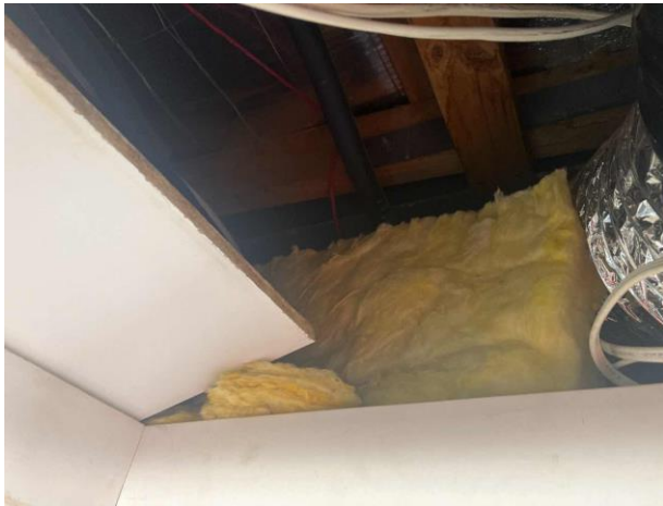
Line ID 168: Internal, Milton Lodge, Accommodation Block, Ceiling Void, Insulation Batts - Suspected SMF
