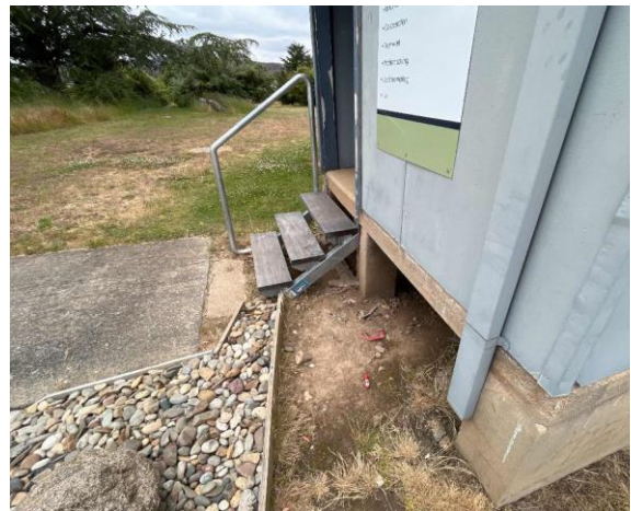
Line ID 40: External, TAFE, Classroom Building, Adjacent Puzzle Room Entry, Ground, Fibre Cement Sheet Debris - Chrysotile & Amosite Asbestos Detected
