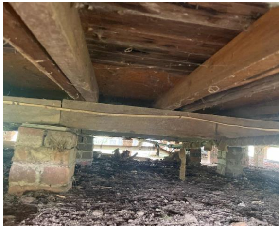
Line ID 47: External, TAFE, Classroom Building, Subfloor, Packers to Columns, Fibre Cement Sheeting - Chrysotile, Amosite and Crocidolite Asbestos Detected
