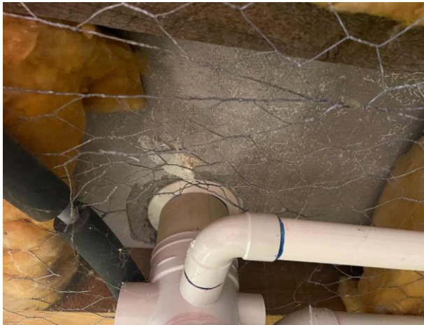
Line ID 135: Internal, Student Lodges, Snowgums Lodge, Basement Plant Room, Ceiling Lining, Compressed Cement Sheeting - Chrysotile Asbestos Detected
