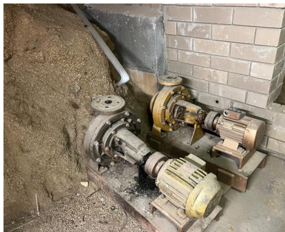
Line ID 112: Internal, Student Lodges, Kareela Lodge, Redundant Plant Equipment, Loose Gasket , Gasket Material - Chrysotile Asbestos Detected
