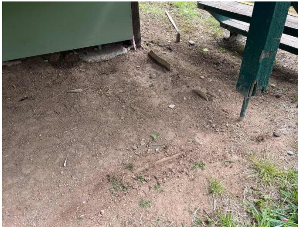
Line ID 16.1: External, Lodge 5, Building Perimeter, West End, Below Deck, in Soil, Fibre Cement Sheet - Chrysotile Asbestos Detected
