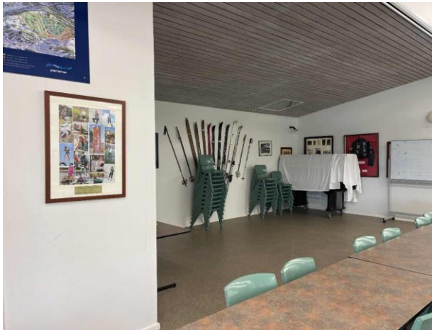
Line ID 76: Internal, Moguls Restaurant, Dining Hall, Display Area, Wall Lining, Fibre Cement Sheet - No Asbestos Detected
