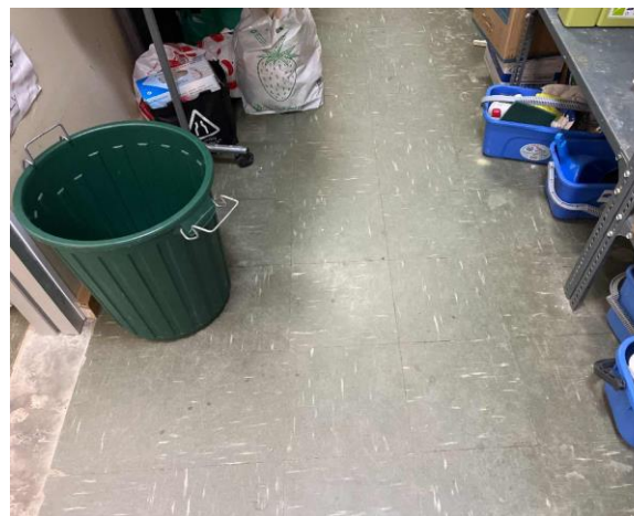
Line ID 67: Internal, Maintenance, Offices and Stores, Floor Covering, Grey Vinyl Floor Tiles - No Asbestos Detected
