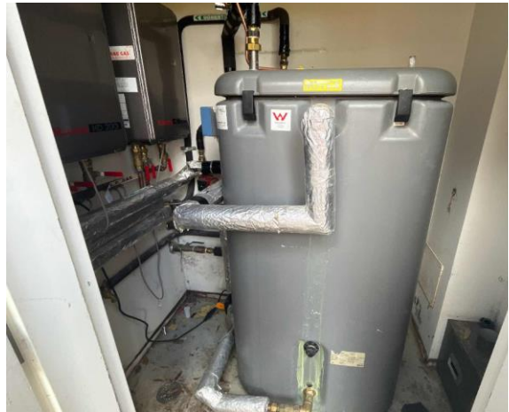
Line ID 170.1: Internal, Milton Lodge, Accommodation Block, Hot Water Unit, Insulation Material - Suspected SMF
