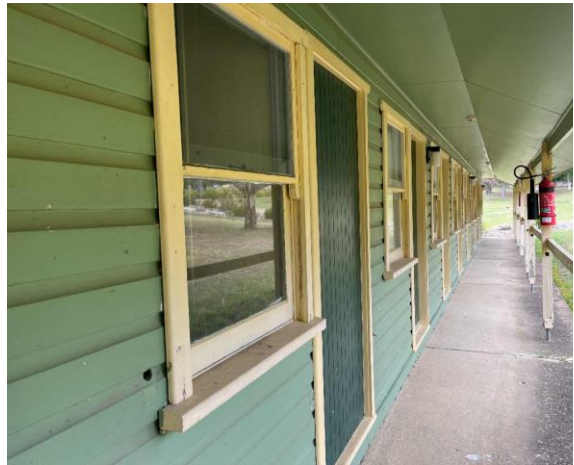
Line ID 148: External, Lodge 5, Veranda, Timber Window Frames, Cream Paint - Lead Detected (36% w/w)
