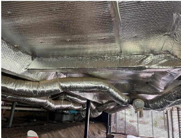
Line ID 153: External, Dining Hall, Subfloor, Ductwork and Sheet Insulation, Insulation Material - Suspected SMF
