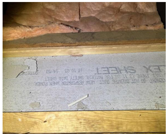
Line ID 55.1: Internal, Lodge 5, Common Room, Wall and Ceiling Lining, Fibre Cement Sheeting - No Asbestos Detected
