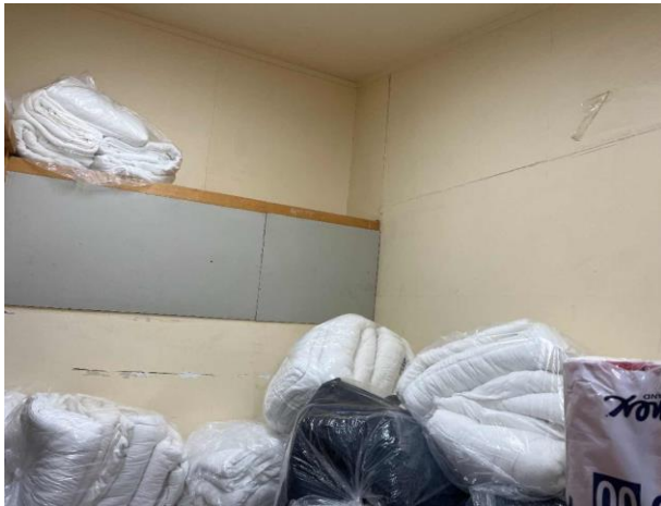
Line ID 63: Internal, Maintenance, Generator Room, Wall Lining, Fibre Cement Sheet - Chrysotile Asbestos Detected
