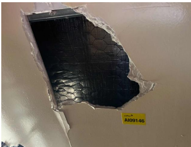
Line ID 78: Internal, Moguls Restaurant, Kitchen, Ceiling Void, Fibre Cement Sheet - No Asbestos Detected
