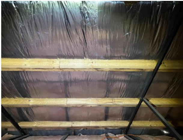
Line ID 163: Internal, Lodge 5, Ceiling Void, Underside of Roof, Sarking Insulation - Suspected SMF
