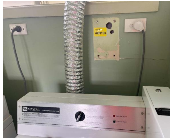
Line ID 58: Internal, Lodge 6, Laundry, Wall Lining, Fibre Cement Sheet - No Asbestos Detected
