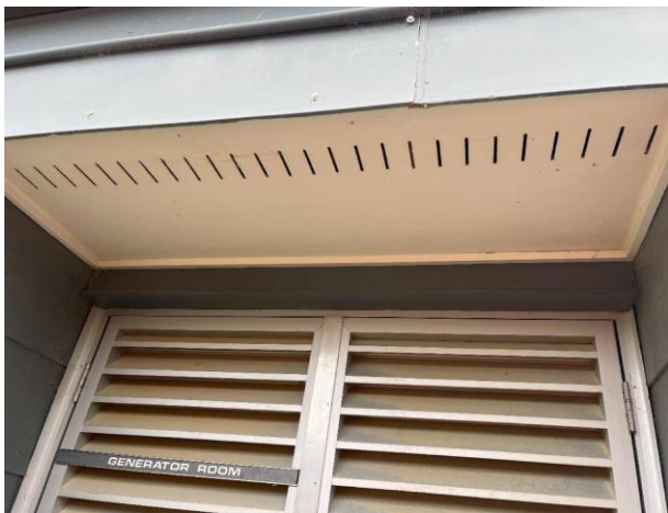
Line ID 25: External, Maintenance, Covered Walkway, Porch Ceiling, Fibre Cement Sheet - Chrysotile Asbestos Detected
