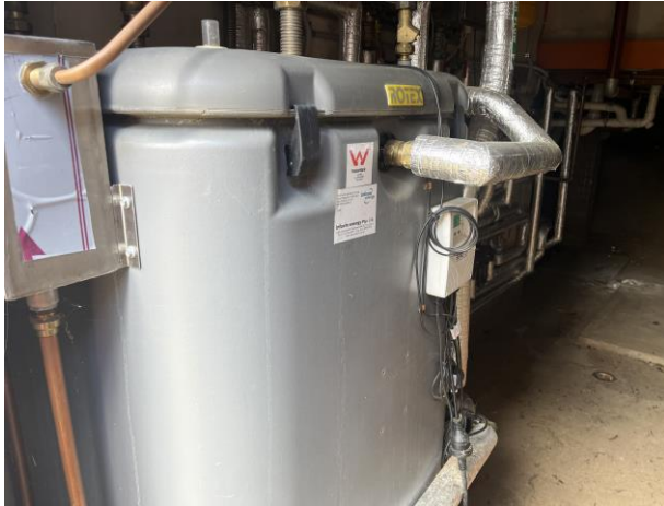
Line ID 188: Internal, Student Lodges, Merritts Lodge, Basement Plant Room, Hot Water Unit, Insulation Material - Suspected SMF
