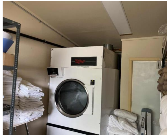
Line ID 66: Internal, Maintenance, Laundry, Wall Lining, Fibre Cement Sheet - Chrysotile Asbestos Detected
