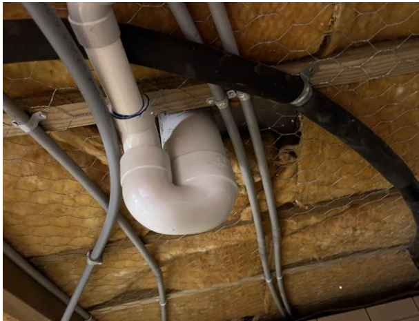
Line ID 190: Internal, Student Lodges, Merritts Lodge, Basement Plant Room, Underside of the Roof, Insulation Batts - Suspected SMF
