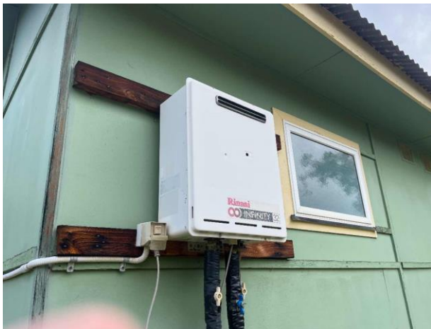
Line ID 154: External, Lodge 5, Toilet Block, Hot Water Unit, Insulation Material - Suspected SMF
