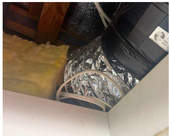
Line ID 167: Internal, Milton Lodge, Accommodation Block, Air Conditioning Ductwork, Insulation Material - Suspected SMF
