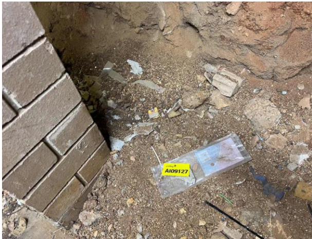
Line ID 134: Internal, Student Lodges, Snowgums Lodge, Basement Plant Room, Adjacent Brick Pillar, Compressed Cement Sheeting Debris - Chrysotile Asbestos Detected
