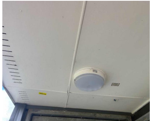
Line ID 24: External, Maintenance, Covered Walkway, Eaves Lining, Fibre Cement Sheet - Chrysotile Asbestos Detected
