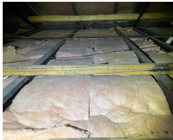
Line ID 162.1: Internal, Lodge 5, Ceiling Void, Throughout, Insulation Batts - Suspected SMF
