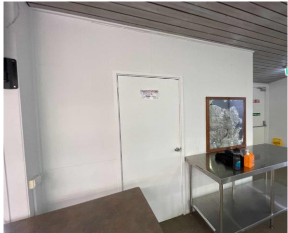
Line ID 77: Internal, Moguls Restaurant, Dining Hall, Storeroom 2, Wall Lining, Fibre Cement Sheet - No Asbestos Detected
