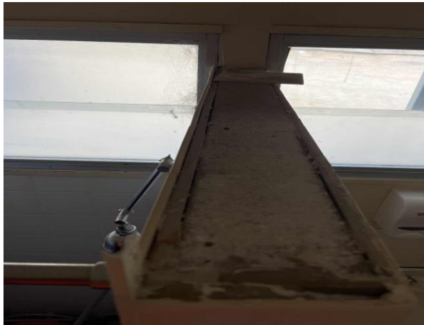
Line ID 68: Internal, Maintenance, Shower and Toilet, Partition Wall, Fibre Cement Sheet - Chrysotile Asbestos Detected
