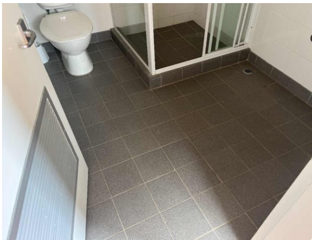
Line ID 140: Internal, Student Lodges, Snowgums Lodge, Level 1, Bathroom and Toilets, Floor Below Ceramic Tiles, Compressed Cement Sheeting - Chrysotile Asbestos Detected
