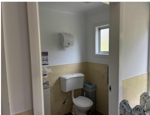
Line ID 72: Internal, Margin Lodge, Laundry & Toilets, Toilets and Laundry, Walls, Fibre Cement Sheet - No Asbestos Detected
