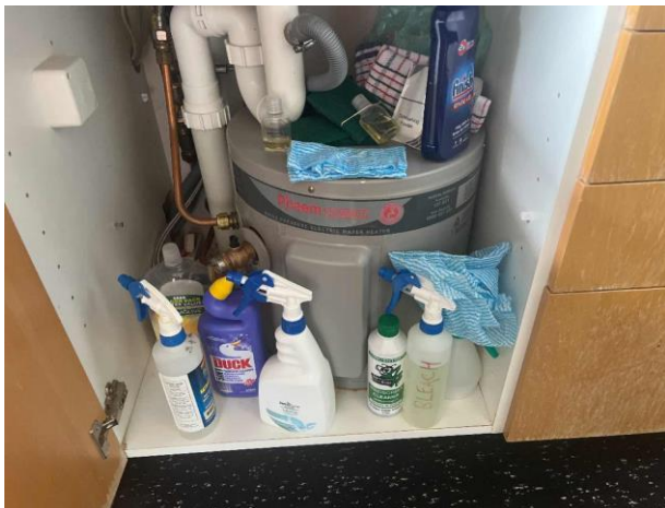
Line ID 175: Internal, Reception, Kitchen, Hot Water Unit, Insulation Material - Suspected SMF
