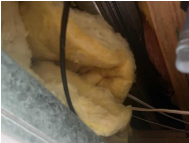
Line ID 173: Internal, Reception, Ceiling Void, Throughout, Insulation Batts - Suspected SMF
