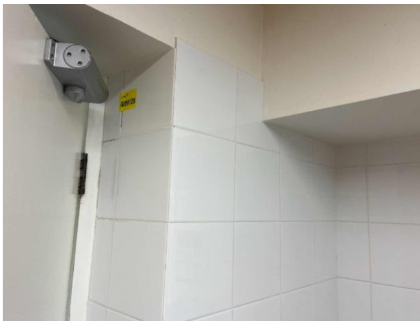
Line ID 143: Internal, Student Lodges, Snowgums Lodge, Toilets, Walls Behind Tiles, Fibre Cement Sheet - No Asbestos Detected
