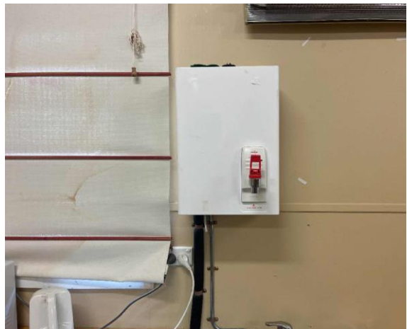
Line ID 201: Internal, TAFE, Classroom, Hot Water Unit, Insulation Material - Suspected SMF
