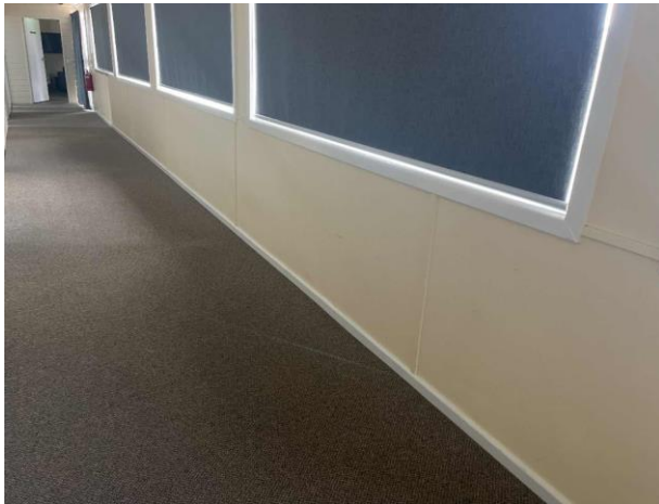
Line ID 70: Internal, Margin Lodge, Corridor, Below Windows, Infill Panels, Fibre Cement Sheet - No Asbestos Detected
