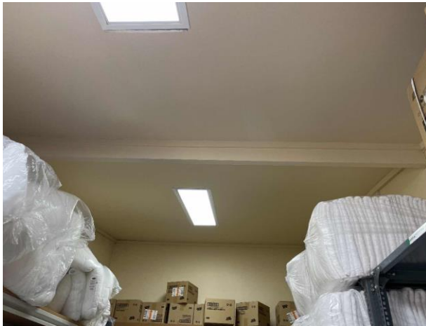
Line ID 65: Internal, Maintenance, Laundry, Ceiling Lining, Fibre Cement Sheet - Chrysotile Asbestos Detected
