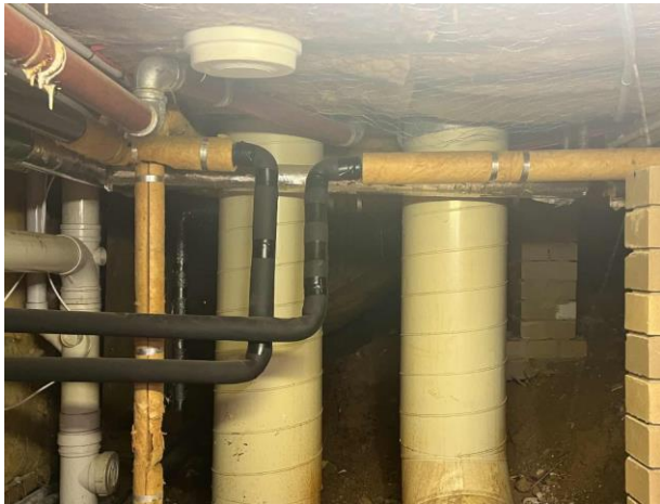
Line ID 198: Internal, Student Lodges, Snowgums Lodge, Basement Plant Room, Pipes, Insulation Material - Suspected SMF
