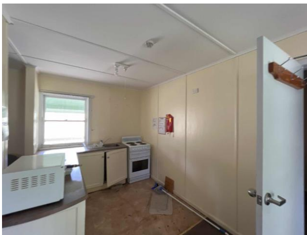
Line ID 55: Internal, Lodge 5, Common Room, Wall and Ceiling Lining, Fibre Cement Sheeting - No Asbestos Detected
