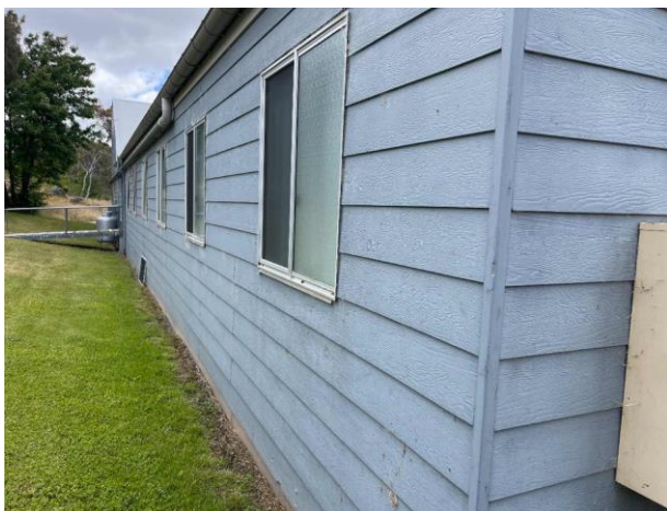
Line ID 27: External, Margin Lodge, Covered Walkways, Walls, Weatherboard Cladding, Fibre Cement Sheet - No Asbestos Detected
