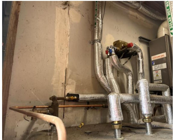
Line ID 117: Internal, Student Lodges, Merritts Lodge, Basement Plant Room, Wall Lining, Fibre Cement Sheet - Chrysotile Asbestos Detected
