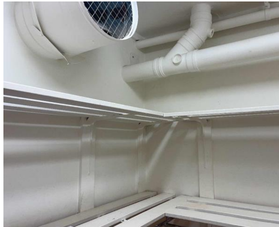
Line ID 139: Internal, Student Lodges, Snowgums Lodge, Drying Room, Wall and Ceiling Lining, Fibre Cement Sheet - No Asbestos Detected
