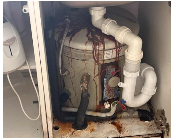
Line ID 164: Internal, Lodge 5, Common Room, Hot Water Unit, Insulation Material - Suspected SMF
