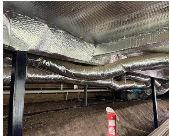
Line ID 153.1: External, Dining Hall, Subfloor, Ductwork and Sheet Insulation, Insulation Material - Suspected SMF
