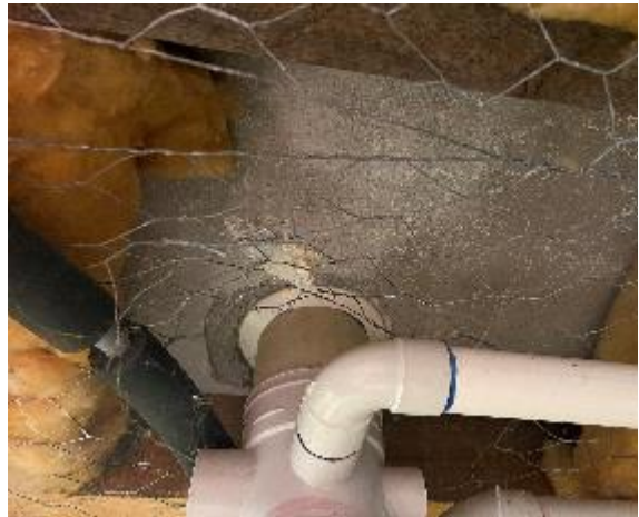
Line ID 115: Internal, Student Lodges, Merritts Lodge, Basement Plant Room, Ceiling Lining, Compressed Cement Sheeting - Chrysotile Asbestos Detected
