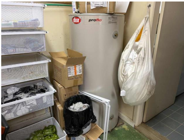
Line ID 165: Internal, Maintenance, Laundry, Hot Water Unit, Insulation Material - Suspected SMF
