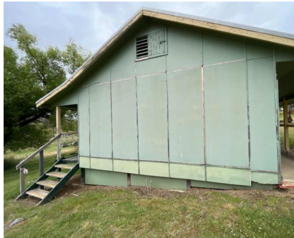
Line ID 14: External, Lodge 5, Building Perimeter, Walls at Building Ends, Fibre Cement Sheet - No Asbestos Detected
