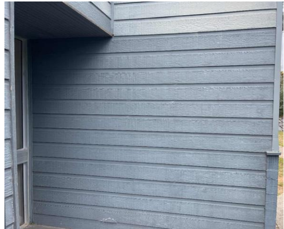
Line ID 38: External, Student Lodges, Snowgums Lodge, Outer Walls, Weatherboard, Fibre Cement Sheet - No Asbestos Detected
