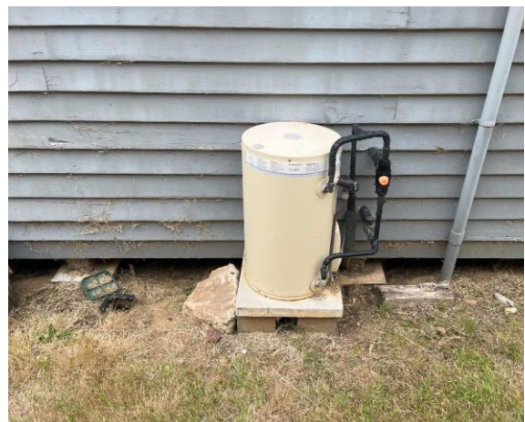
Line ID 157: External, TAFE, Classroom Building, Hot Water Unit, Insulation Material - Suspected SMF
