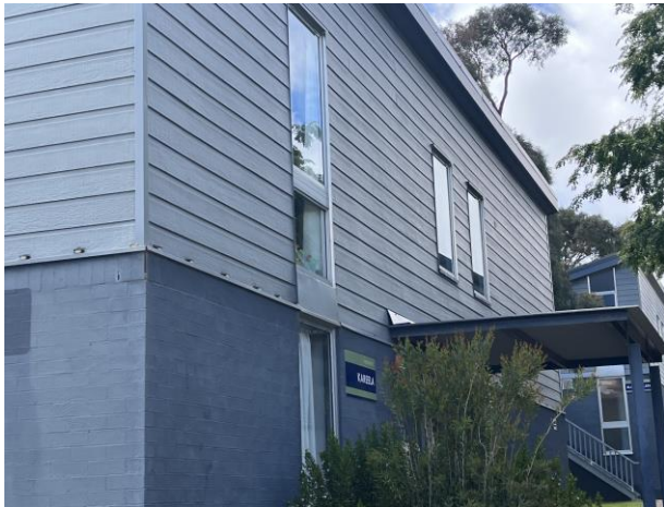
Line ID 32: External, Student Lodges, Kareela Lodge, Outer Walls, Weatherboard, Fibre Cement Sheet - No Asbestos Detected
