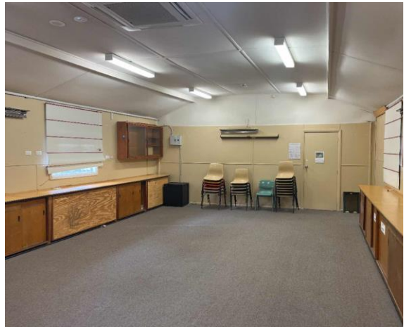
Line ID 150: Internal, TAFE, Classroom, Walls, Cream Paint - Lead Detected (0.33% w/w)
