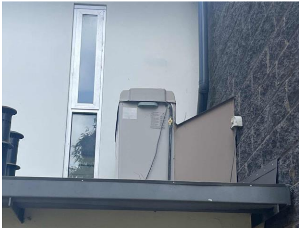
Line ID 170: Internal, Milton Lodge, Accommodation Block, Hot Water Unit, Insulation Material - Suspected SMF
