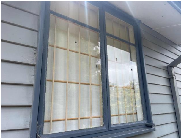
Line ID 49: External, TAFE, Classroom Building, Window Frames, Window Caulking - Chrysotile Asbestos Detected
