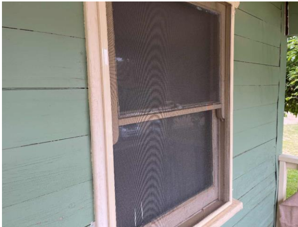
Line ID 22: External, Lodge 6, Rear Standalone House, Window Frames, Window Caulking - No Asbestos Detected
