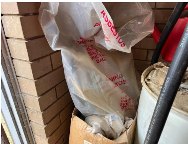
Line ID 61: Internal, Maintenance, Chemical Store, Waste Bag of Asbestos Adjacent Entry Door, Fibre Cement Sheet - Suspected Asbestos
