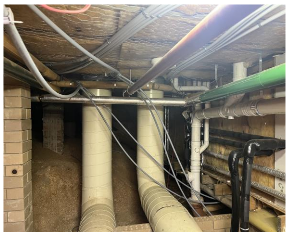
Line ID 185: Internal, Student Lodges, Kareela Lodge, Basement Plant Room, Pipes, Insulation Material - Suspected SMF
