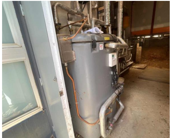
Line ID 197: Internal, Student Lodges, Snowgums Lodge, Basement Plant Room, Hot Water Unit, Insulation Material - Suspected SMF
