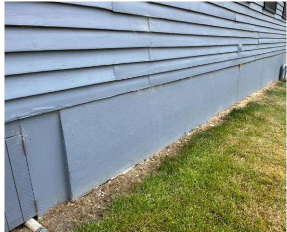
Line ID 51: External, Torino Lodge, Rear Lower Section to Subfloor, Low Level Panels, Fibre Cement Sheet - No Asbestos Detected
