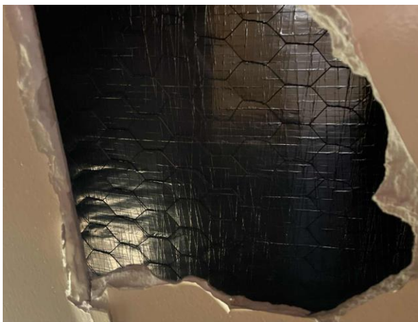
Line ID 171: Internal, Moguls Restaurant, Kitchen, Ceiling Void, Underside of Roof, Sarking Insulation - Suspected SMF
