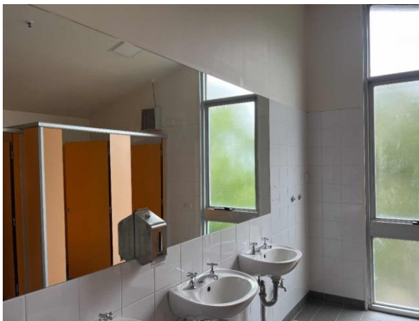
Line ID 141: Internal, Student Lodges, Snowgums Lodge, Level 1, Toilets, Walls Behind Tiles, Fibre Cement Sheet - No Asbestos Detected
