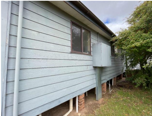
Line ID 44: External, TAFE, Classroom Building, North East Area, Weatherboard, Fibre Cement Sheet - No Asbestos Detected
