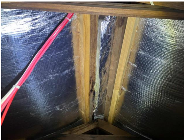
Line ID 200: Internal, TAFE, Toilets, Ceiling Void, Underside of Roof, Sarking Insulation - Suspected SMF
