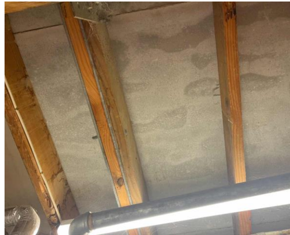
Line ID 136: Internal, Student Lodges, Snowgums Lodge, Basement Plant Room, High Ceiling Lining, Compressed Cement Sheeting - Chrysotile Asbestos Detected
