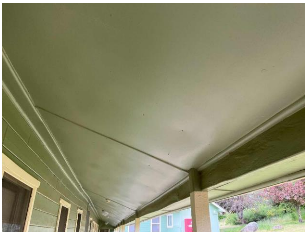
Line ID 20: External, Lodge 6, Accommodation Block, Eave and Veranda Ceiling, Fibre Cement Sheet - No Asbestos Detected
