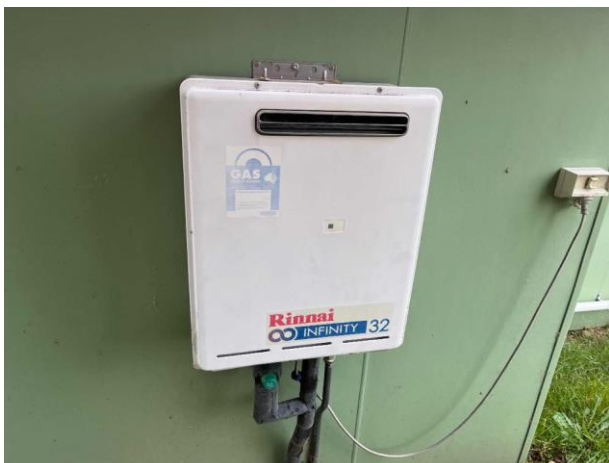
Line ID 156: External, Lodge 6, Guest Laundry, Hot Water Heater, Insulation Material - Suspected SMF
