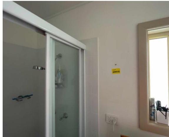
Line ID 60: Internal, Lodge 6, Rear Standalone House, Toilet and Shower, Wall Lining, Fibre Cement Sheet - No Asbestos Detected
