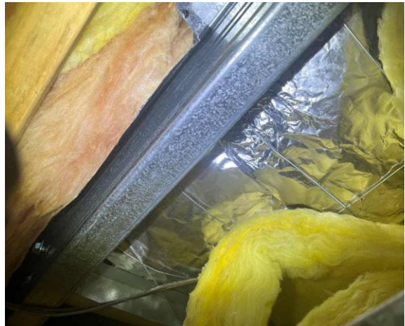
Line ID 174: Internal, Reception, Ceiling Void, Underside of Roof, Sarking Insulation - Suspected SMF
