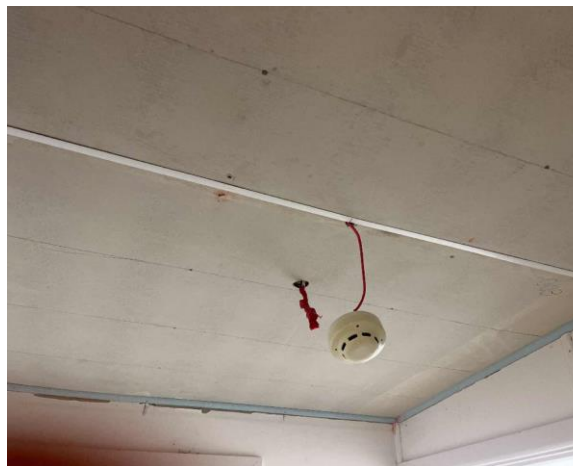
Line ID 144: Internal, TAFE, Toilets, Porch Entry, Ceiling Lining, Fibre Cement Sheet - No Asbestos Detected
