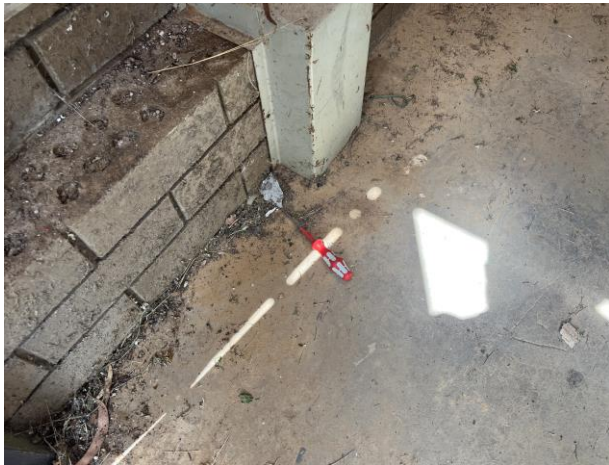
Line ID 114: Internal, Student Lodges, Merritts Lodge, Basement Plant Room, Adjacent Brick Pillar, Compressed Cement Sheeting Debris - Chrysotile Asbestos Detected
