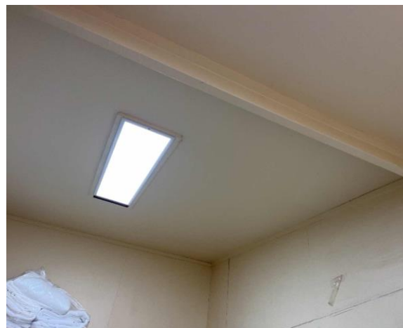
Line ID 62: Internal, Maintenance, Generator Room, Ceiling Lining, Fibre Cement Sheet - Chrysotile Asbestos Detected
