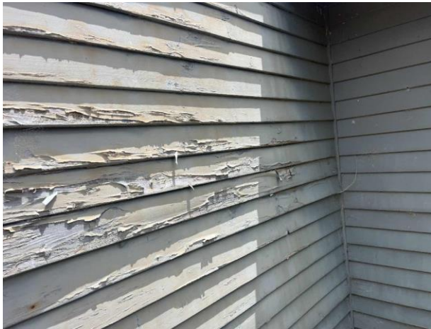
Line ID 149: External, TAFE, Classroom Building, Timber Walls, Light Green Paint - Lead Detected (5.5% w/w)
