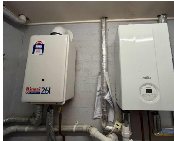
Line ID 161: Internal, Conference Centre, Boiler Room, Hot Water Unit, Insulation Material - Suspected SMF
