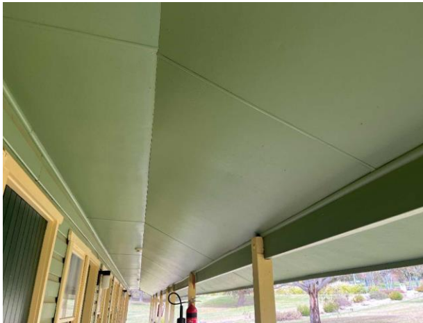
Line ID 18: External, Lodge 5, Veranda, Eave and Ceiling Lining, Fibre Cement Sheet - No Asbestos Detected
