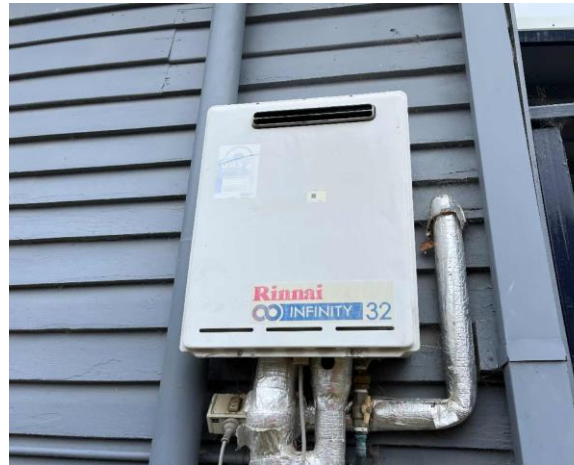
Line ID 159: External, Torino Lodge, Rear Lower Section to Subfloor, Hot Water Units, Insulation Material - Suspected SMF
