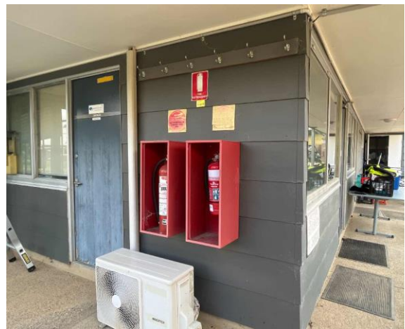
Line ID 26: External, Maintenance, Covered Walkway, Wall Panels, Fibre Cement Sheet - Chrysotile Asbestos Detected
