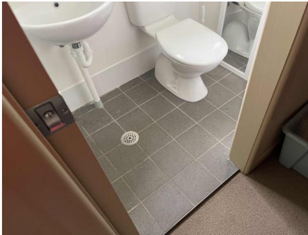
Line ID 59: Internal, Lodge 6, Rear Standalone House, Bathroom, Below Ceramic Tiles to Floor, Compressed Cement Sheet - Suspected Asbestos
