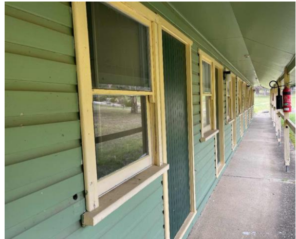
Line ID 19: External, Lodge 5, Veranda, Timber Windows, Window Caulking - No Asbestos Detected
