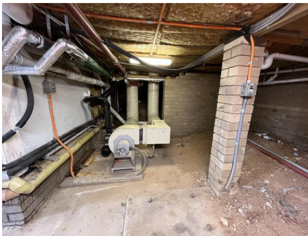
Line ID 124: Internal, Student Lodges, Ramshead Lodge, Basement Plant Room, Adjacent Brick Pillar, Compressed Cement Sheeting Debris - Chrysotile Asbestos Detected
