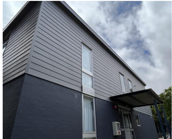
Line ID 34: External, Student Lodges, Merritts Lodge, Outer Walls, Weatherboard, Fibre Cement Sheet - No Asbestos Detected
