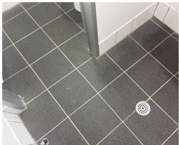
Line ID 82: Internal, Reception, Toilets, Below Ceramic Tiles to Floor, Compressed Cement Sheet - Suspected Asbestos
