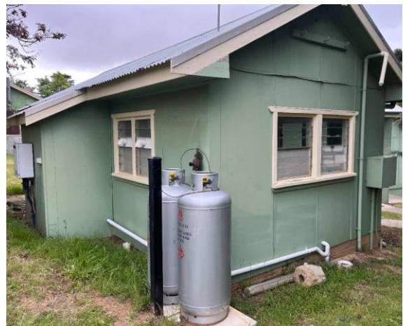
Line ID 21: External, Lodge 6, Guest Laundry, Wall Lining, Fibre Cement Sheet - Chrysotile, Amosite and Crocidolite Asbestos Detected
