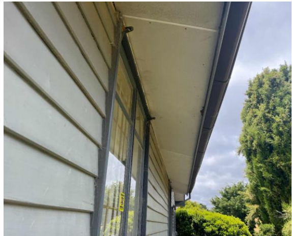
Line ID 41: External, TAFE, Classroom Building, Eaves, Fibre Cement Sheet - No Asbestos Detected
