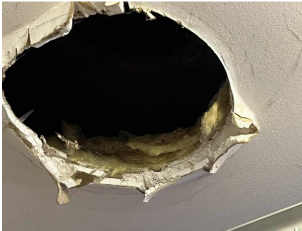
Line ID 160: Internal, Conference Centre, Boiler Room, Ceiling Void, Insulation Batts - Suspected SMF
