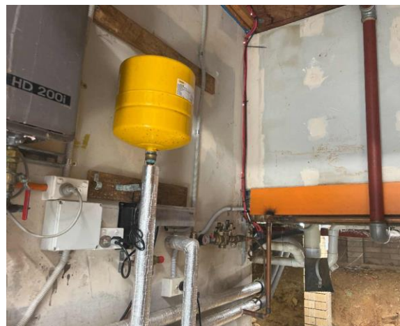
Line ID 137: Internal, Student Lodges, Snowgums Lodge, Basement Plant Room, Wall Lining, Fibre Cement Sheet - Chrysotile Asbestos Detected
