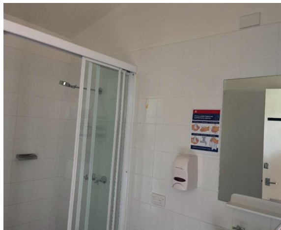
Line ID 141.1: Internal, Student Lodges, Snowgums Lodge, Level 1, Toilets, Walls Behind Tiles, Fibre Cement Sheet - No Asbestos Detected
