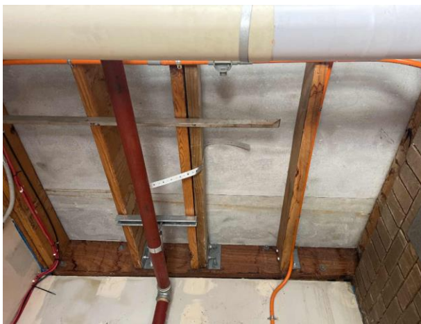
Line ID 136.1: Internal, Student Lodges, Snowgums Lodge, Basement Plant Room, High Ceiling Lining, Compressed Cement Sheeting - Chrysotile Asbestos Detected
