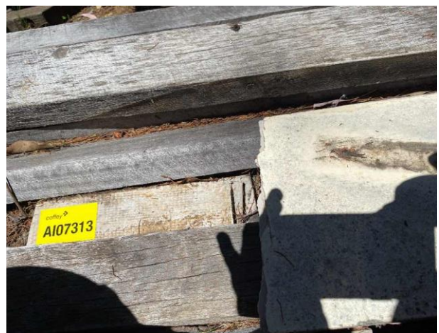
Line ID 32: External, Maintenance Shed, East Elevation, Amongst Timber Work, Debris, Fibre Cement Sheet - Chrysotile and Amosite Asbestos Detected
