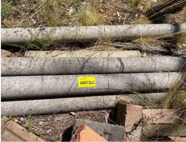
Line ID 33: External, Maintenance Shed, East Elevation, Stored Pipework Adjacent Old Equipment, Moulded Fibre Cement - Chrysotile, Amosite and Crocidolite Asbestos Detected
