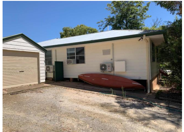
Line ID 53: External, Private Residence B, House Perimeter, Eave Lining, Fibre Cement Sheet - Chrysotile, Amosite, and Crocidolite Asbestos Detected
