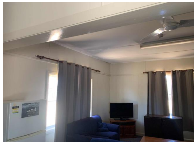
Line ID 85: Internal, Kilpara, Kitchen, Wall and Ceiling Linings, Fibre Cement Sheet - Chrysotile Asbestos Detected
