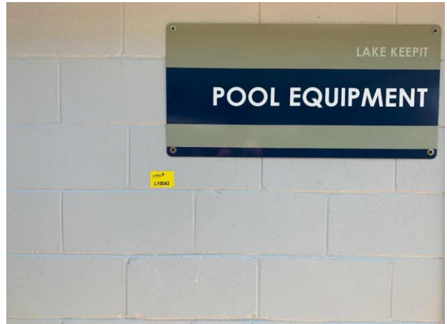
Line ID 139: External, Pool Pump House, Throughout, Walls, Off White Paint - Lead Detected (<0.005% w/w)
