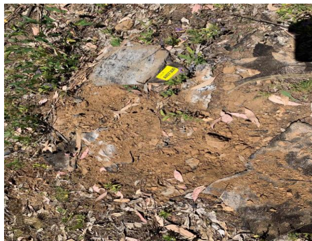
Line ID 31: External, Maintenance Shed, Debris Throughout, West Adjacent to Storage Shelves, Bituminous Material - No Asbestos Detected
