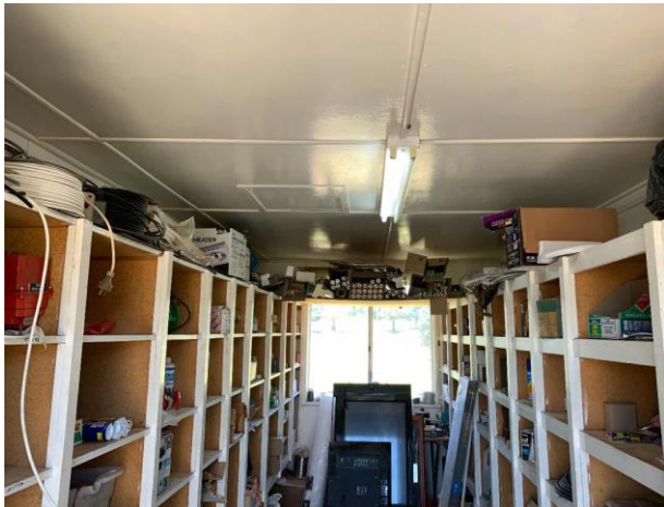
Line ID 119: Internal, Workshop, South Store, Walls and Ceiling, Fibre Cement Sheet - Chrysotile Asbestos Detected
