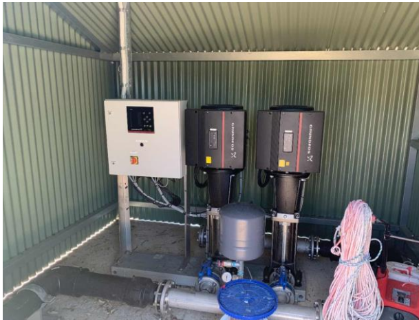
Line ID 113: Internal, Water Treatment Shed, , South Wall, Compressed Cement Sheet - Removed
