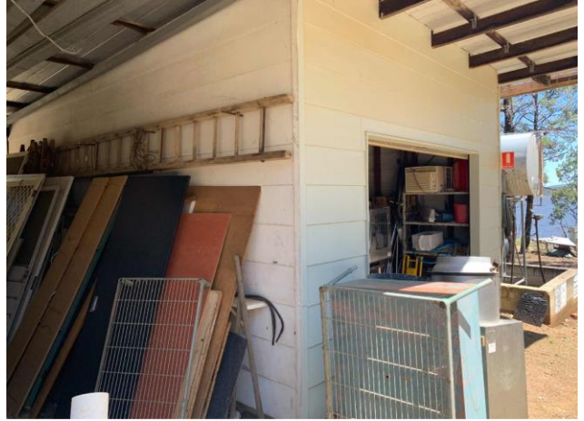
Line ID 34: External, Maintenance Shed, Garage Storeroom, Weatherboard Cladding and Joinery, Fibre Cement Sheet - Chrysotile & Amosite Asbestos Detected
