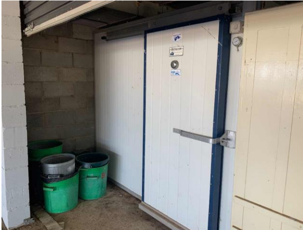
Line ID 151: Internal, Dining Hall, Basement, Refrigeration Unit, Internal Insulation - Suspected SMF
