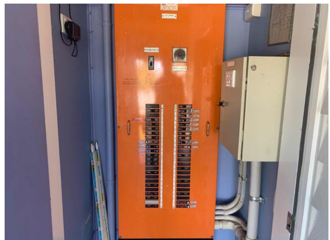
Line ID 144: Internal, Lodges Inc. Dilapidated Toilet Block, Block A, Within Services Closets, Purple Paint - Lead Detected (0.03% w/w)
