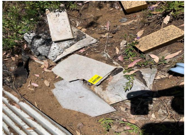
Line ID 30: External, Maintenance Shed, Debris Throughout, West Adjacent to Storage Shelves, Compressed Cement Sheet - Chrysotile Asbestos Detected
