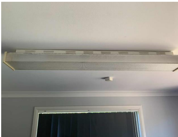
Line ID 111: Internal, Staff Quarters and Accommodation, Girls Toilets North of New Extension, Wall Linings, Fibre Cement Sheet - Chrysotile Asbestos Detected
