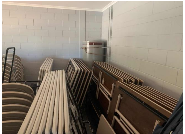
Line ID 154: Internal, Homestead, Throughout, Chair Storage Room, Hot Water Heater, Internal Insulation - Suspected SMF
