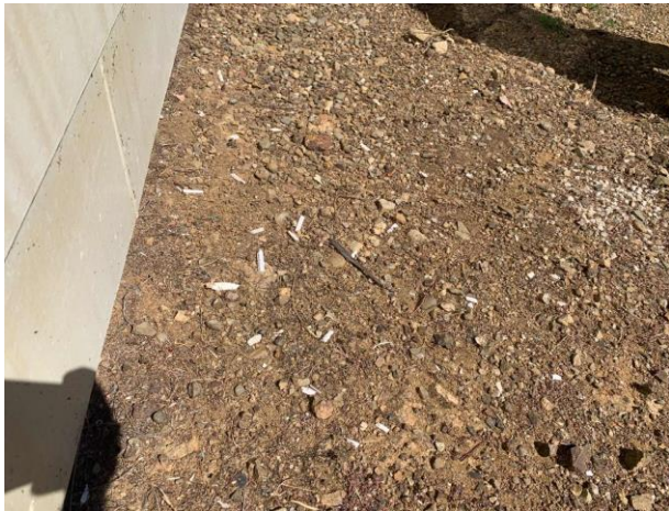
Line ID 21: External, Hilltop Lodge, Throughout, East Elevation, Debris, Window Caulking - No Asbestos Detected
