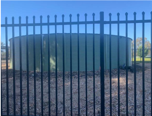
Line ID 65: External, Water Treatment Shed, Water Tank, Southeast Face, Panelling, Resinous Electrical Backing Board - No Asbestos Suspected
